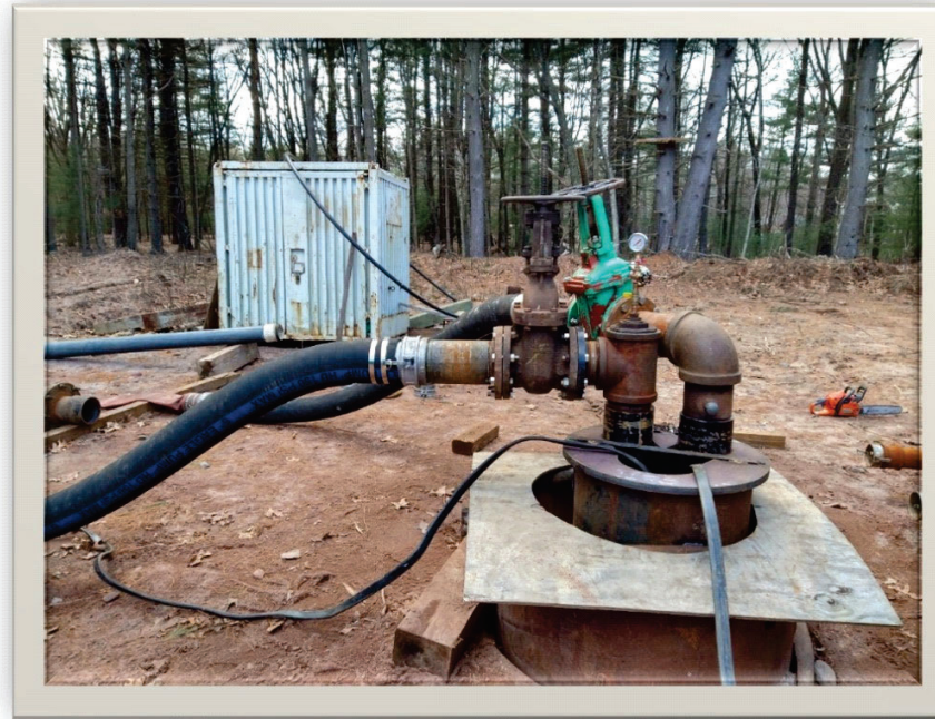
Well # 10 Pump Test Photo
